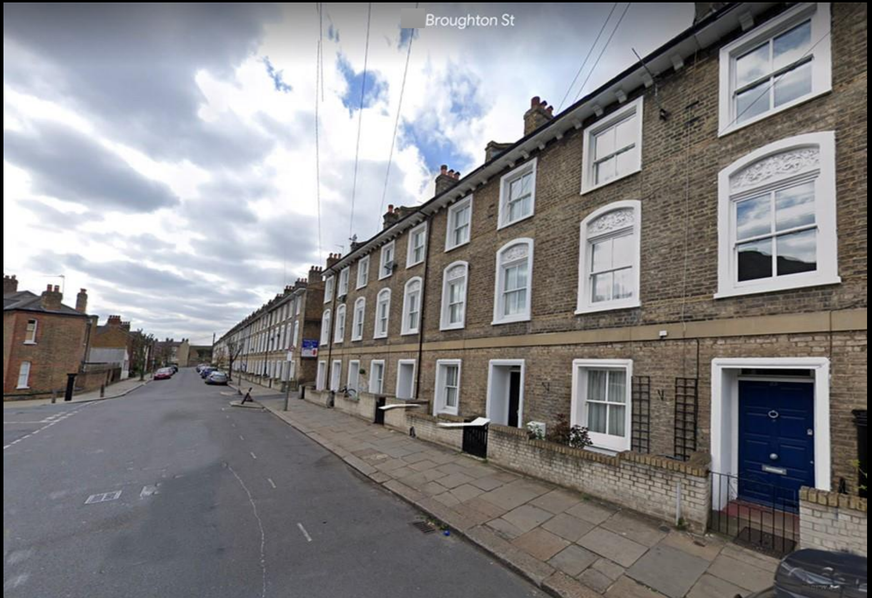
Broughton Street, Battersea today. No. 24 is the house with the blue door on the right.
